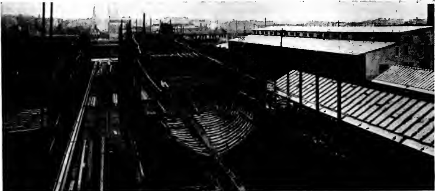
General view of the two building slips, now occupied with vessels, showing handling space between hulls.
